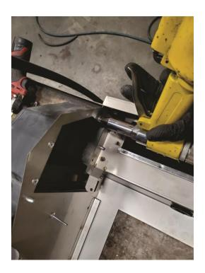
2. Install a gasket for the fresh air intake.
